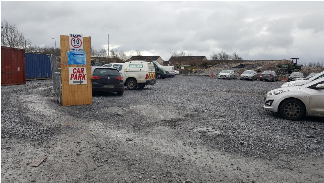
Plate 11-6: Hardcore surfaced carpark within construction compound which occupies southern half of the eastern portion of the proposed development site.
