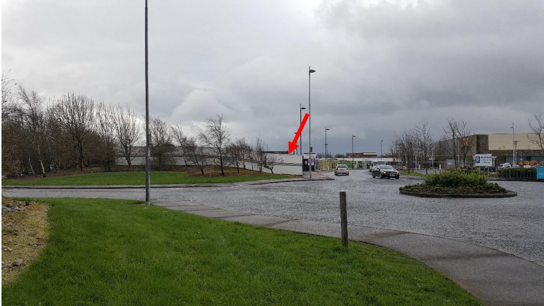
Plate 11-5: Access road currently dividing the eastern portion of the proposed development site, looking south towards construction compound (arrow).
