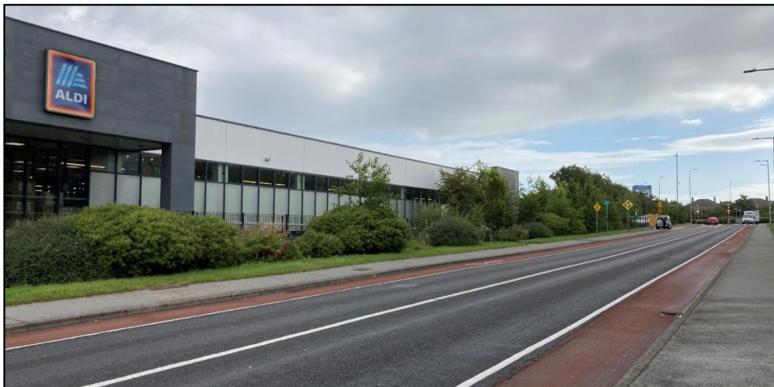
Plate 12-11 View north from the Western Distributor Road beside the ALDI Supermarket
